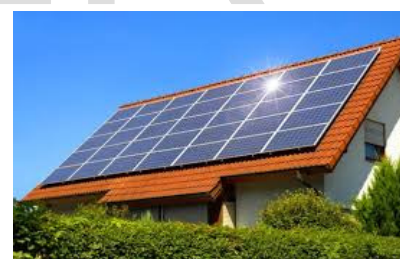
Fig. 4 Rooftop Building Management System
